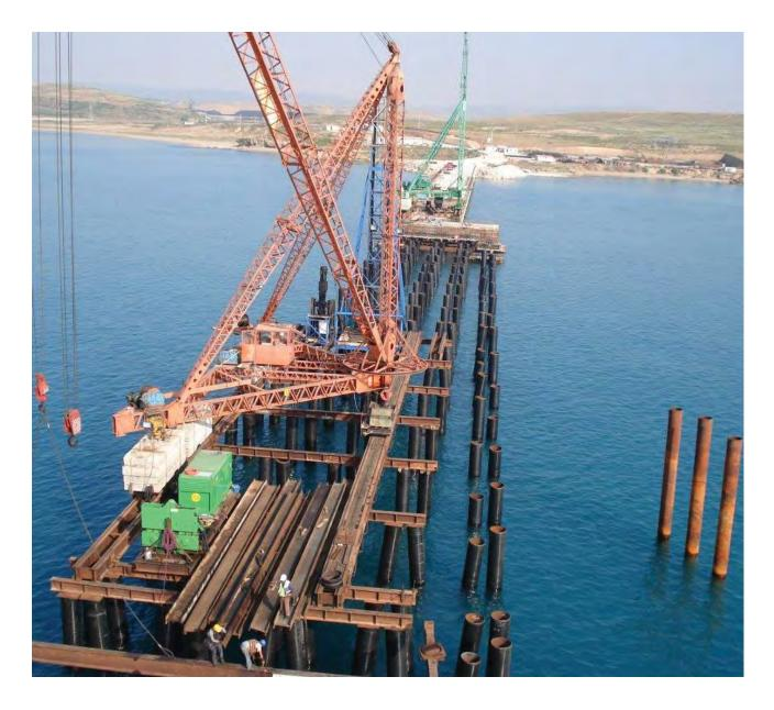
Piles are one of the major components of most marine structures. KDI has vast experience within the field of offshore piledriving owing to kilometers of pile installations under varying circumstances.
